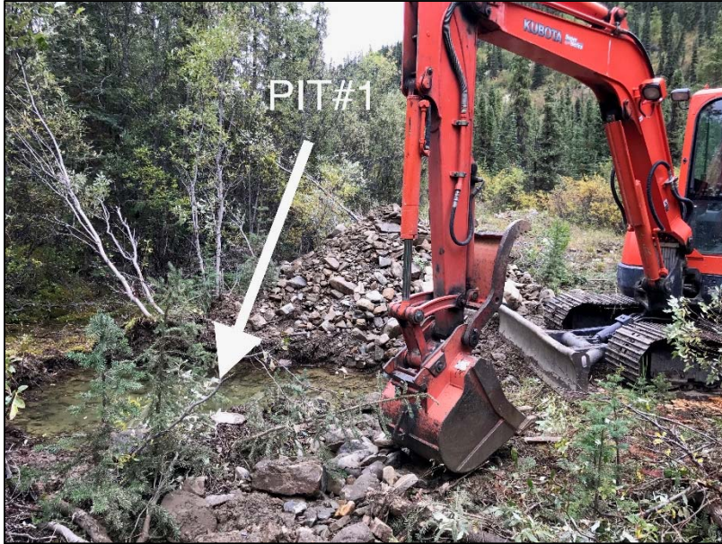
Figure 11 Pit # 1 and Excavator
