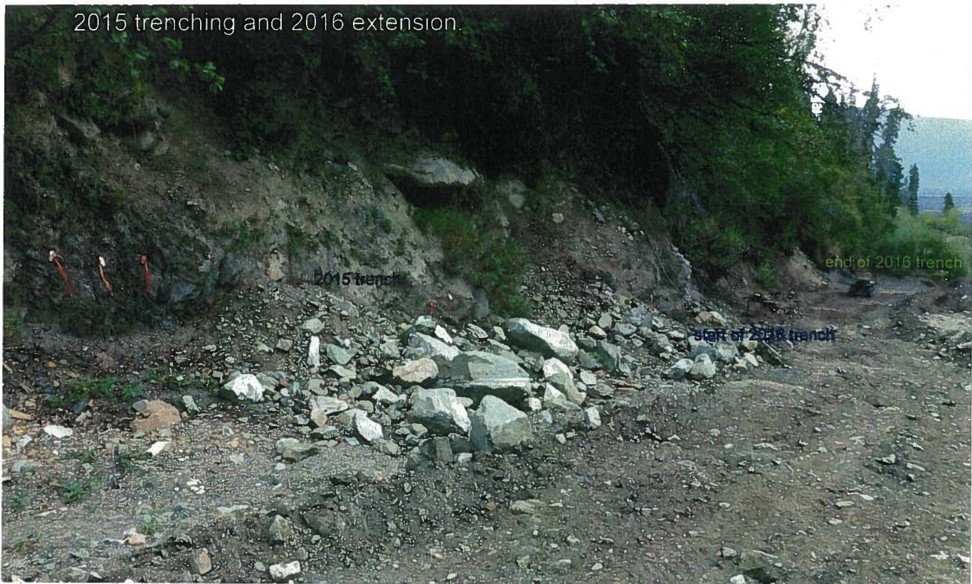
Photo 4: 2015 bulldozer trench and 80 metre – 2016 extension on Left Limit
