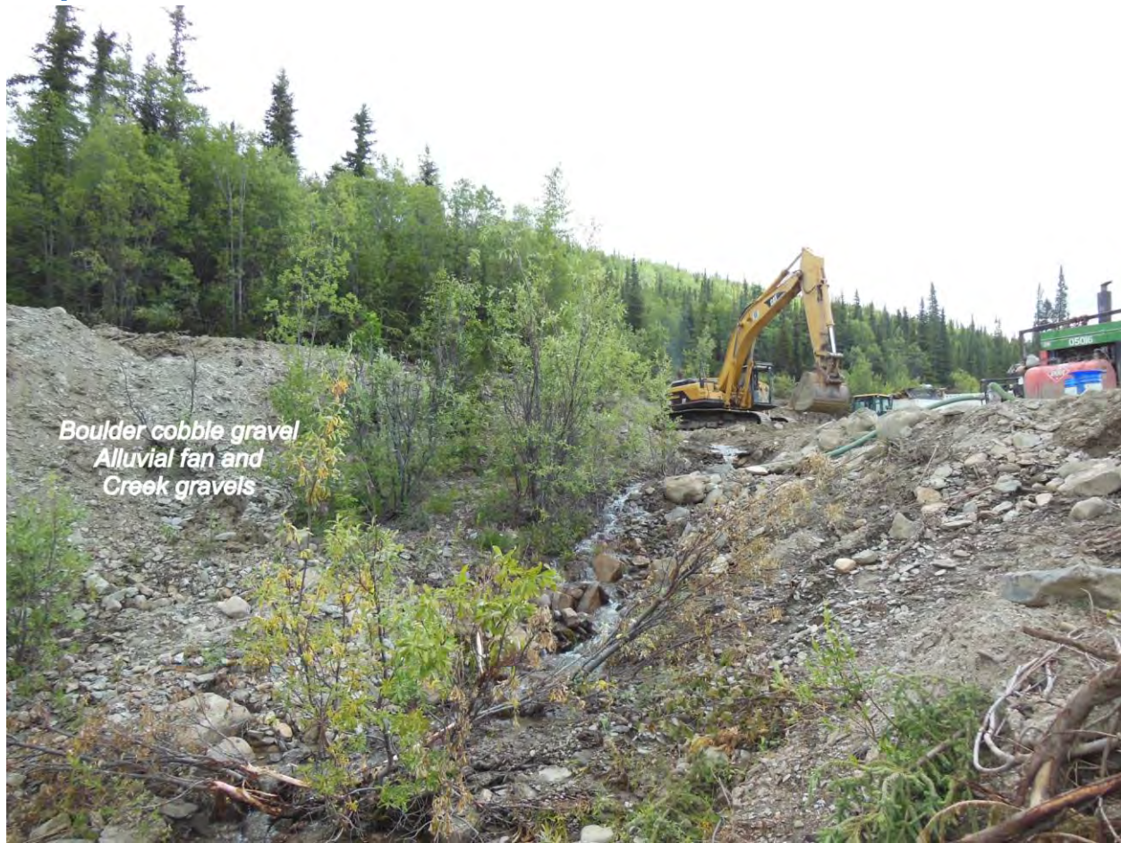
Figure 20 - Test Pit 2016-02 was excavated in a creek channel within the alluvial fan. This pit was excavated approximately 25 feet into boulder cobble creek and alluvial fan gravels.
