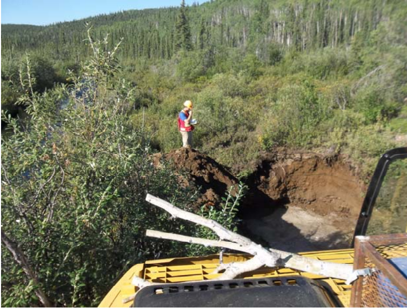
Photo 2. Test pit at the junction of Meloy Creek and Casino Creek
