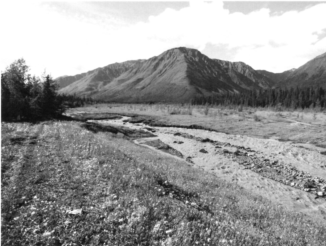
Plate 1 - View of Nines Creek looking upstream at the spillway channel, which usually is not occupied by water. The access road was washed out at this point.
