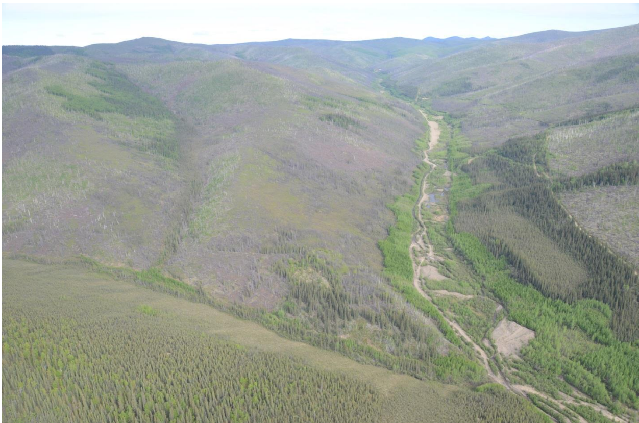
Plate 1- View looking north (upstream) on Maisy May Creek at the confluence with Patton Creek, June 2013. Patton Creek in mid-foreground joins Maisy May Creek from the left side of the photo.
