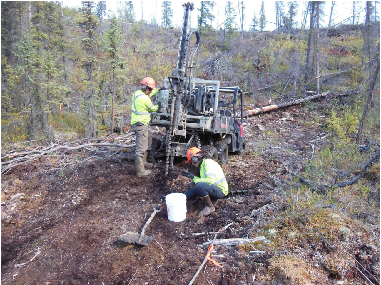
Plate 5 - Auger drilling on Patton Creek tributary Mila Creek, on resistivity line PC A.
