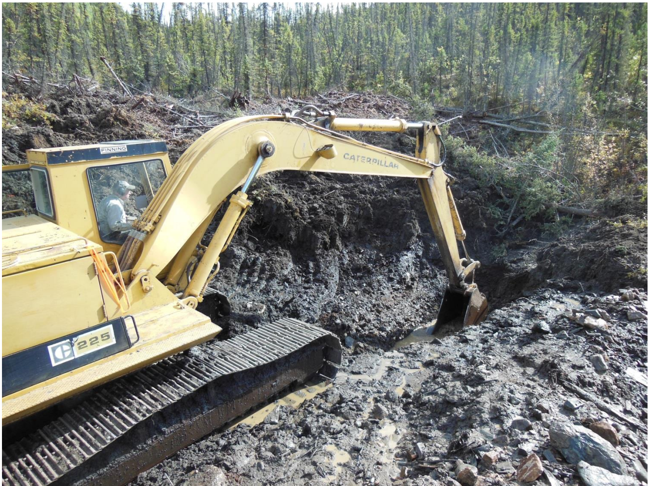
Plate 5 - Caterpillar 225 excavator operated by Bud Davis at test-pit CAN 14-01.
