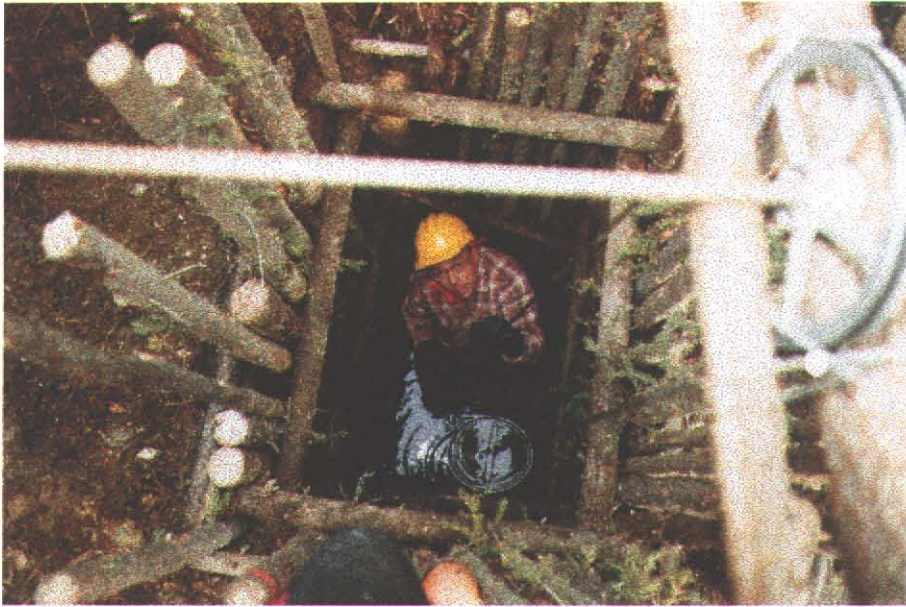
Peter Malacarne bailing water from Shaft #2
