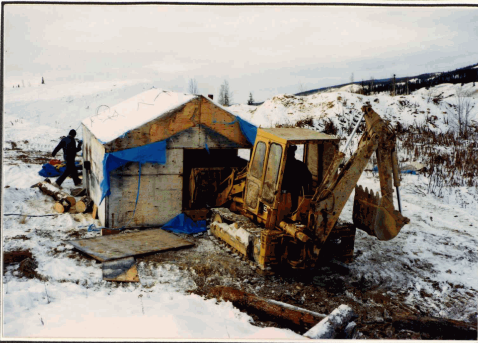
6A. Caterpillar 931 Traxcavator dumping first sample into processing shack. Tailings chute of Spriggs Jig shows on left wall of shack.
