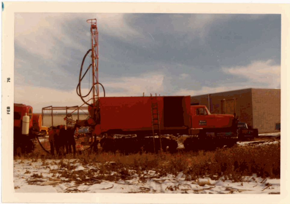
Plate I : View of the Foremost 8T. The drill is set-up for work with the compressor to the left on the Nodwell.
