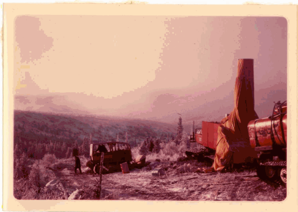
Plate III : A view down Discovery Creek showing all the equipment. The caterpillar D6C is on the left. The drill is shown with the special cover used for winter drilling.
