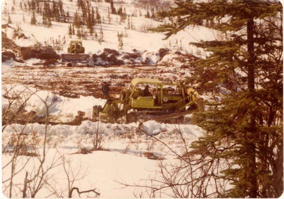
Start of construction of the upper storage dam on Kenyon Creek. April 1976.
