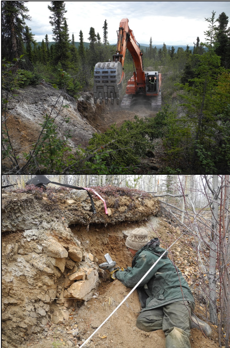
Figure 6.3: Upper image shows deepening old trenches in Zone A in 2015 with an excavator. Lower image shows an XRF being used to delineate sample intervals in a Zone B trench that has been cleaned by hand.
