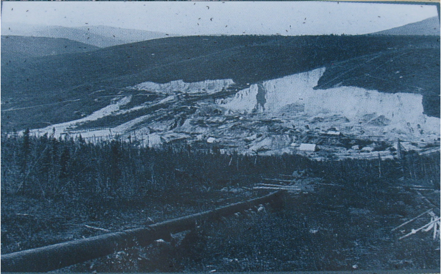
Picture from the ridge road heritage trail depicting Cripple Hill roughly a century ago. These two white channel hills have been mined continually since the beginning of the gold rush more than 100 years ago and are still producing gold today, out of the gravels and along the hard rock horizon, as well as out of decomposing exposed bedrock beneath the discarded overburden.
