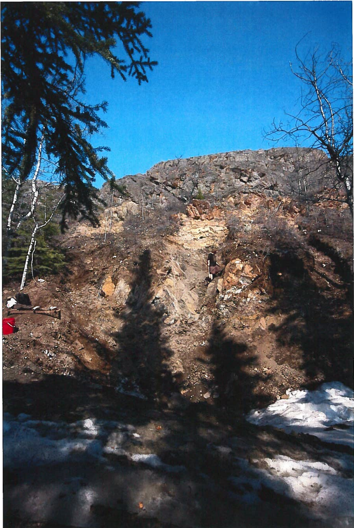
Main Zone Trenching 2012
