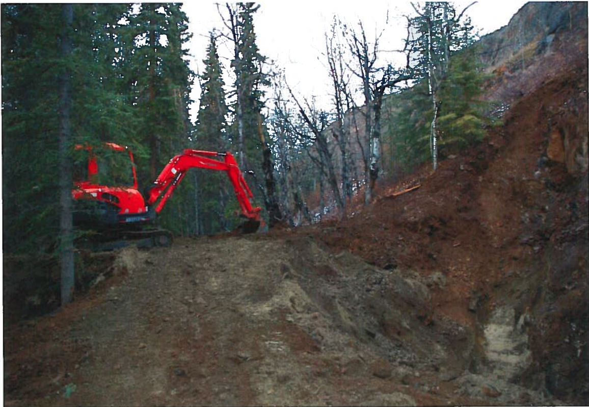
Reclamation at Main Zone with KX121-3 Excavator
