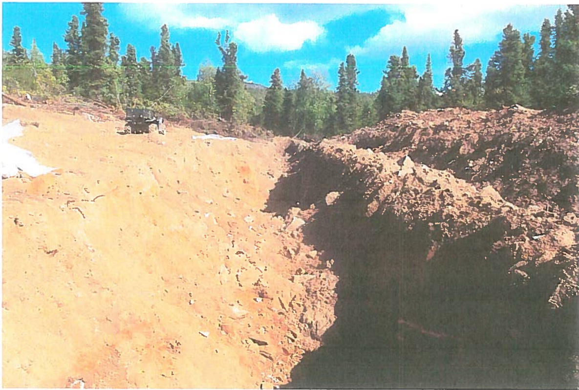
Photo 4: Trenching at the SB zone. Sample series SB-2 is in the foreground. SB-3 is mid picture
