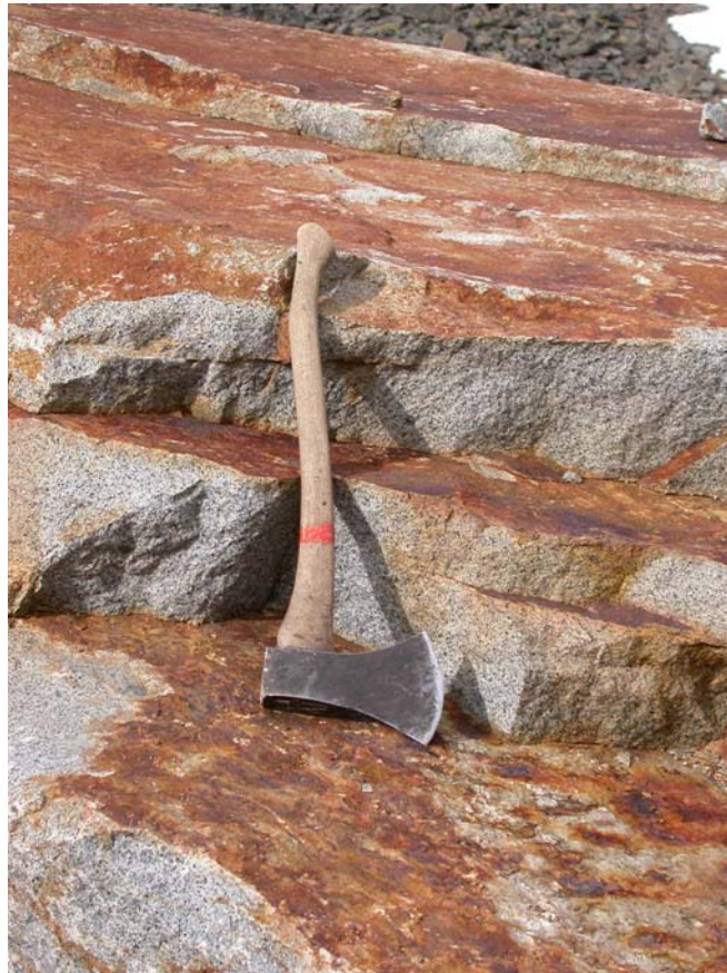
Rusty dry fracture
