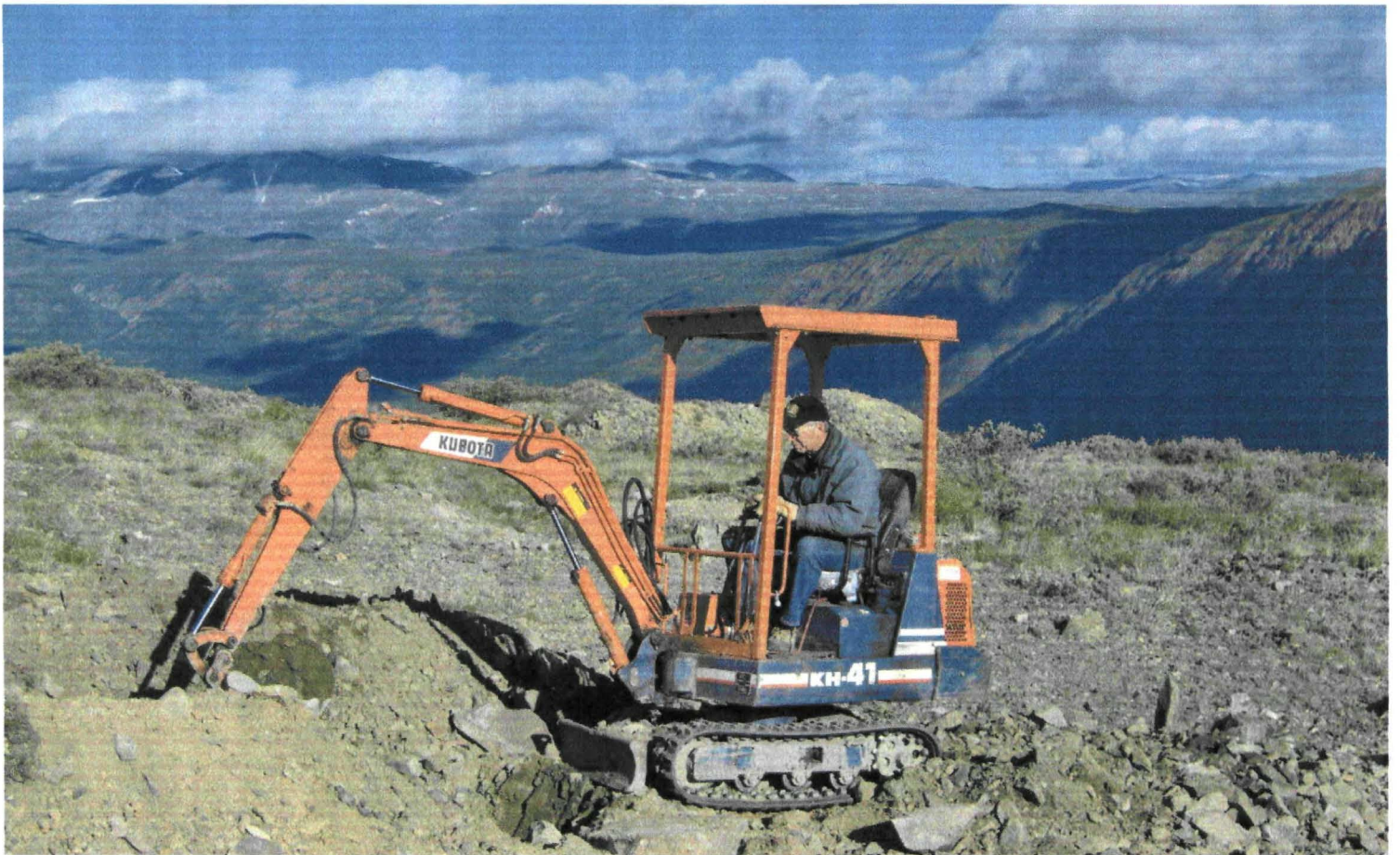
TRENCHING ON THE EAST ZONE RED RIDGE PROPERTY - AUGUST 2007
