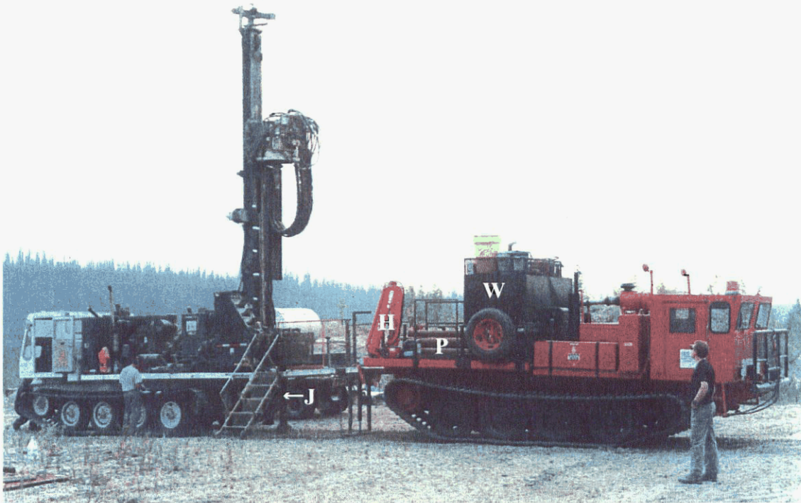
Plate 1b - Overview of the rig showing the the belt-tracked drilling and support Nodwells parked back-to-back and joined by a working platform. Note the hydraulic leveling jacks (J) under the drilling Nodwell and the drill pipe (P), hydraulic hoist (H) and water tank (W) on the support Nodwell.
