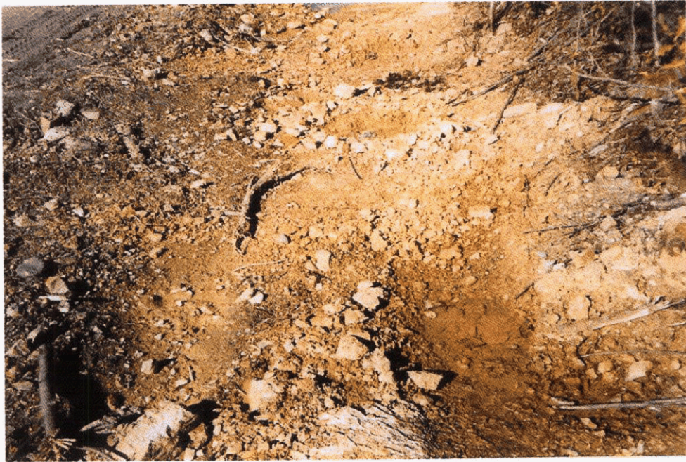
Excavated Trench at 3ACE road outcrop
