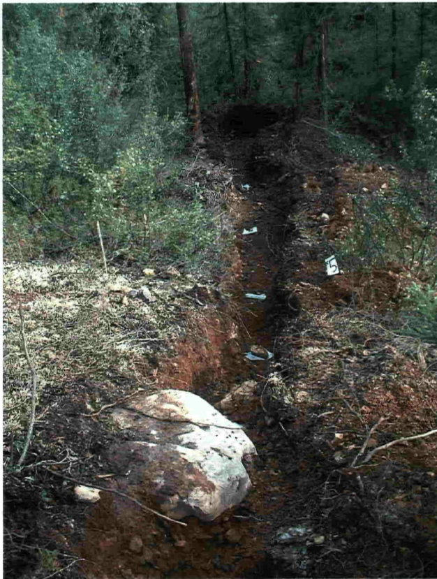
Photo 13. North part of Trench 5.
