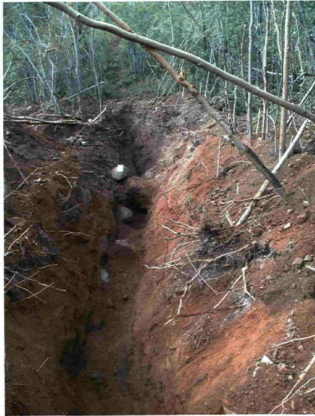
Photo 3. South end of Trench 1.
