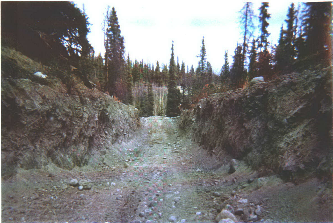
Photo 1 Excavated Trench on PROTECTOR 3, looking due East.
