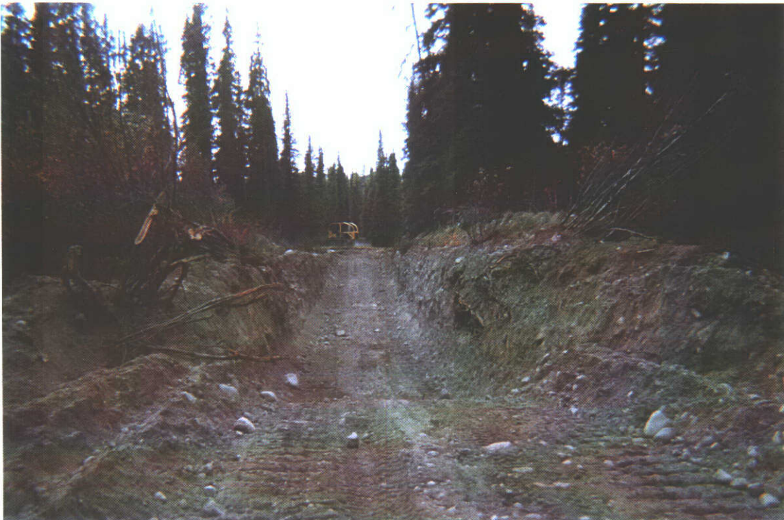
Photo 2: Excavated Trench on PROTECTOR 3, looking due West.
