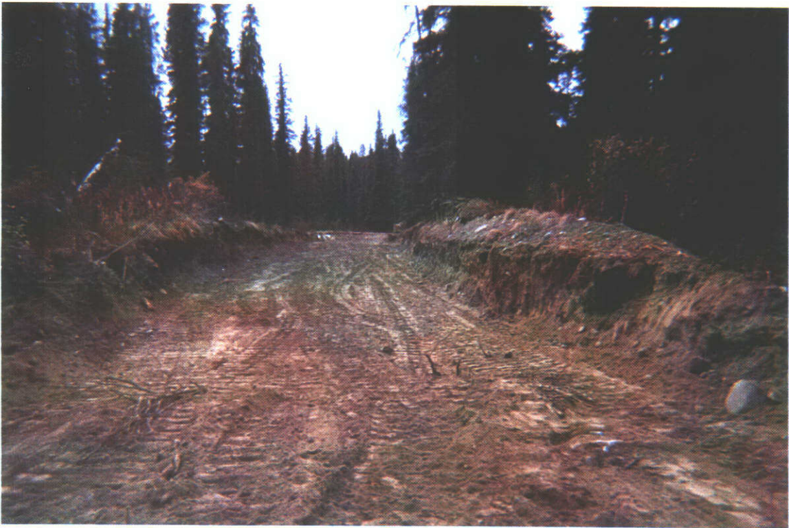
Photo 4: Reclaimed Trench on PROTECTOR 3, looking due West.
