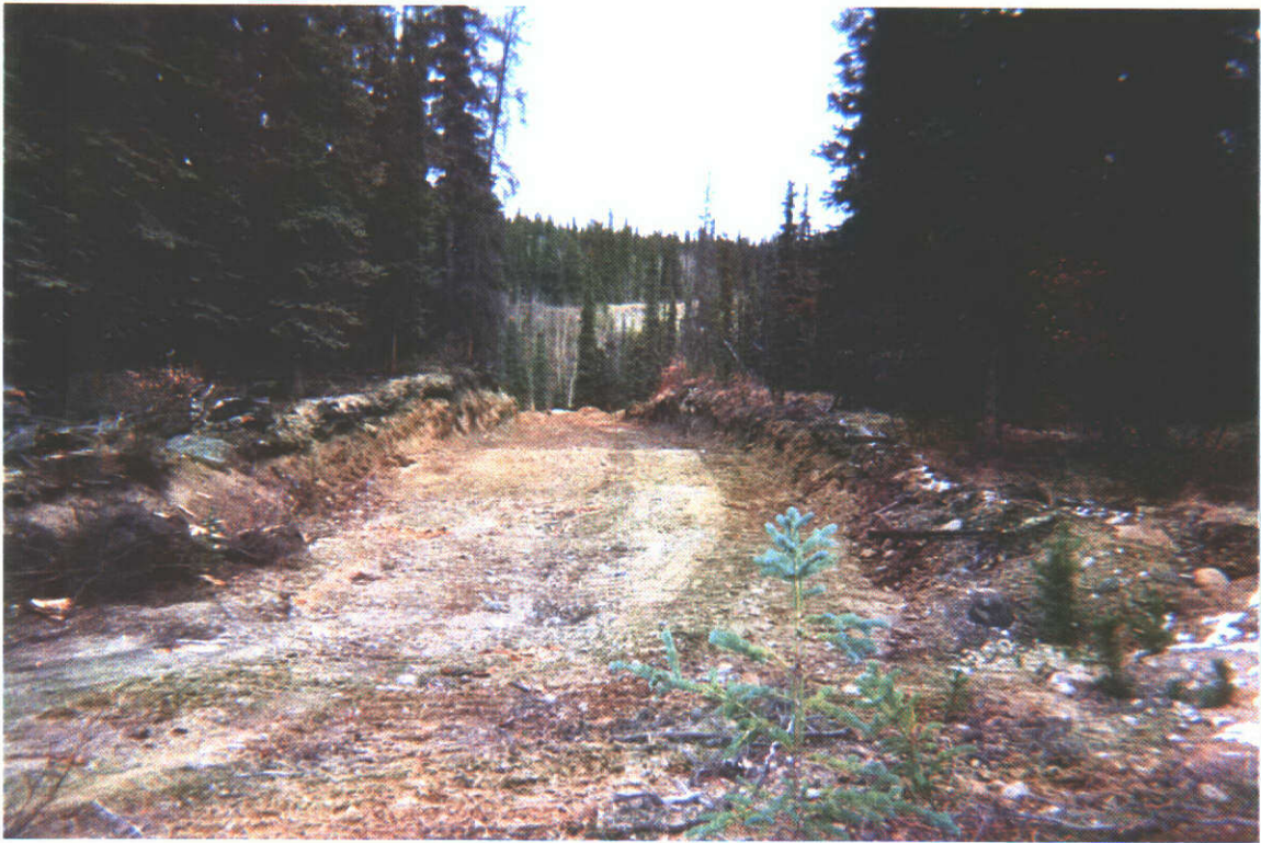
Photo 3 Reclaimed Trench on PROTECTOR 3, looking due East.
