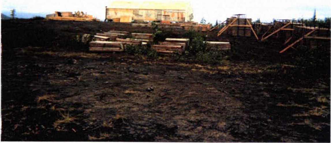
Photo 1, Ice Property – Camp, core racks and kitchen building
