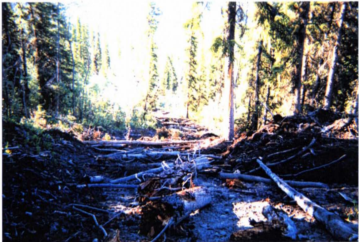
Photo 8, Ice Property – Access road to lower pump
