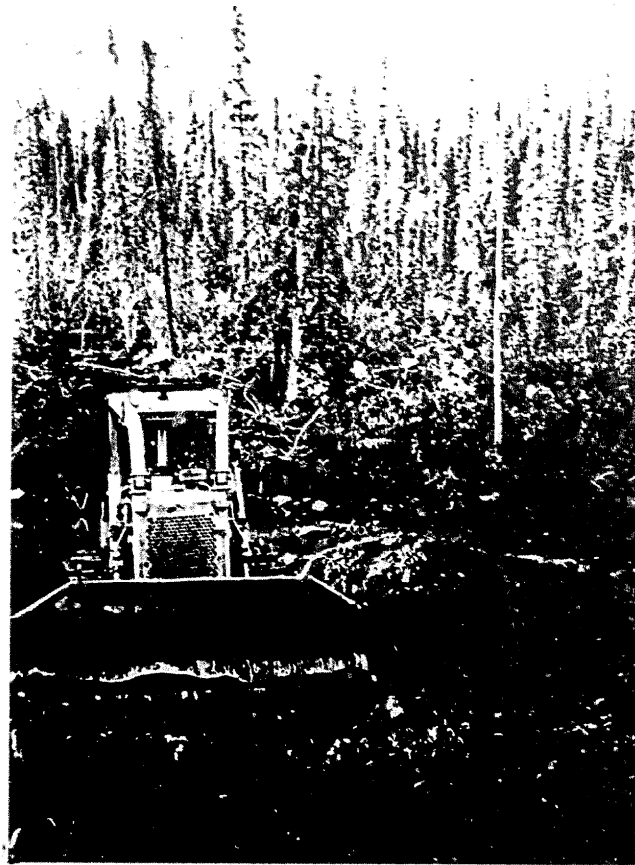
Stripping vegetation covering and insulating permafrost in placer creek.
