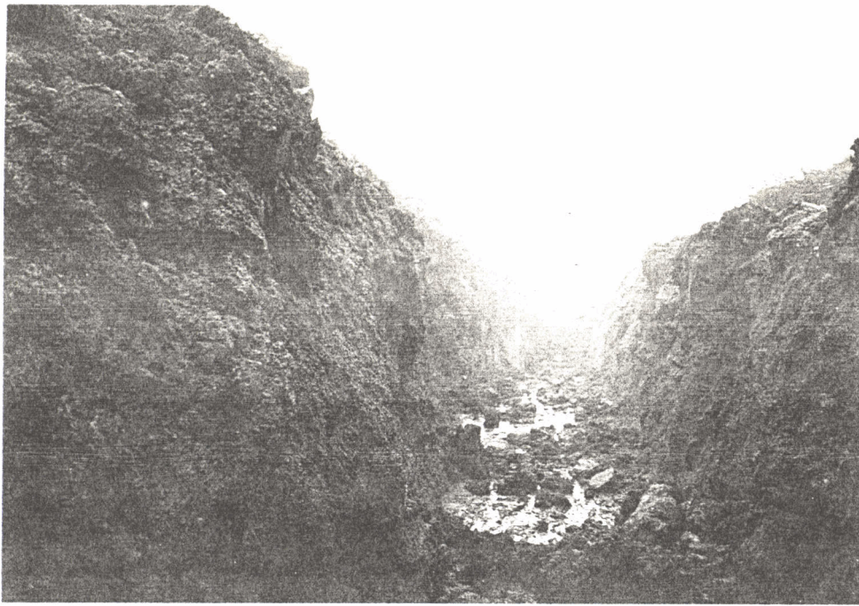
Trenching to bedrock through thawed ground.
