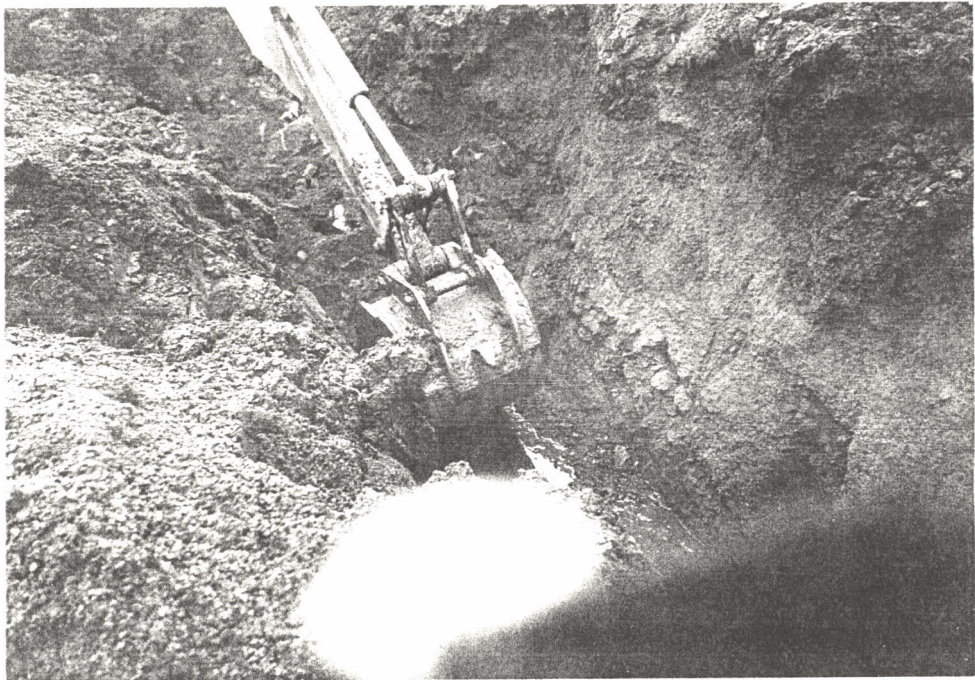
Backhoe trenching decomposed in-situ bedrock. Vein and wallrock alteration dipping at 30^\circ can be seen to the lower right of backhoe bucket.
