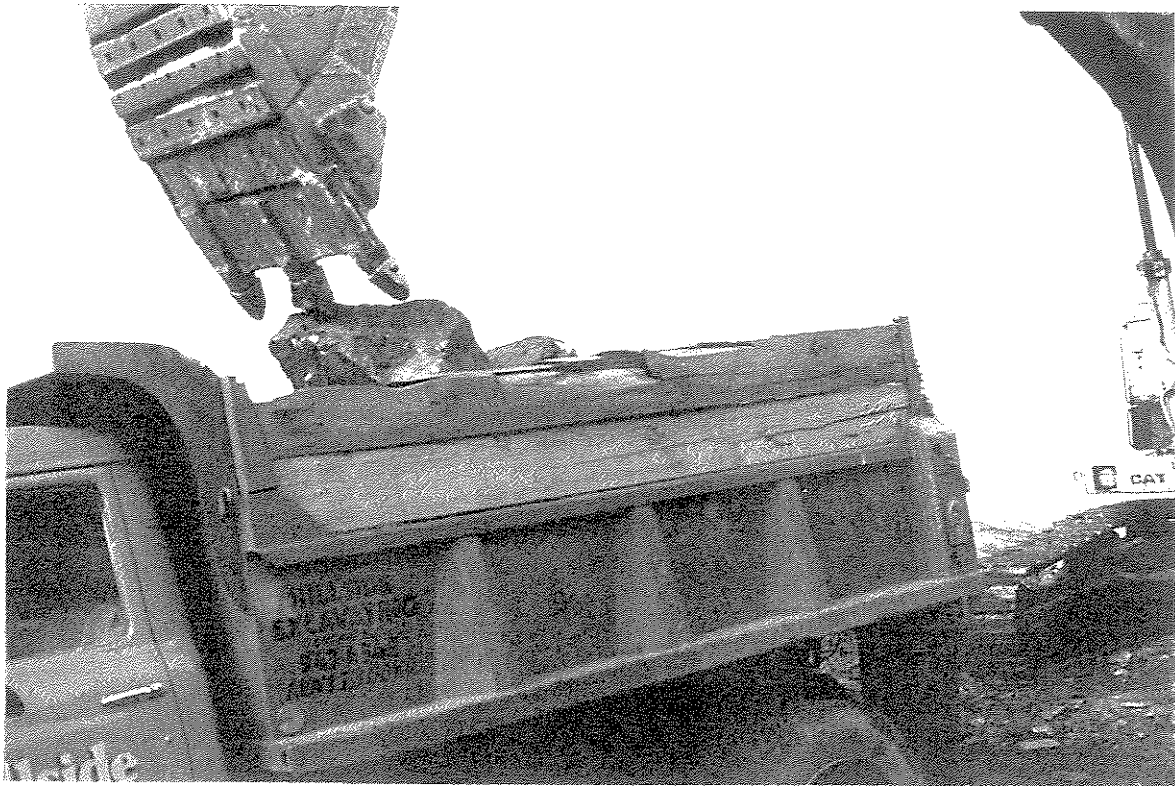
Loading dump truck.
