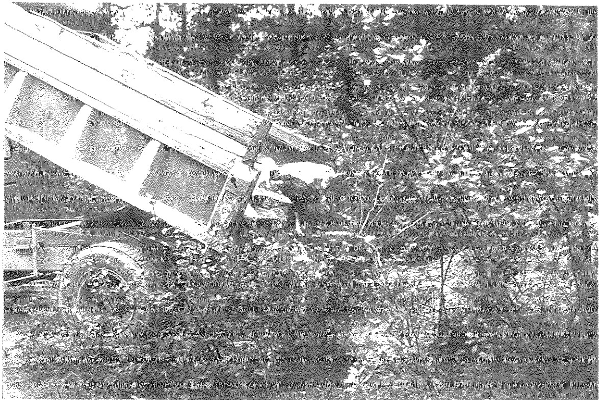
Dumping at Camol Road staging area.
