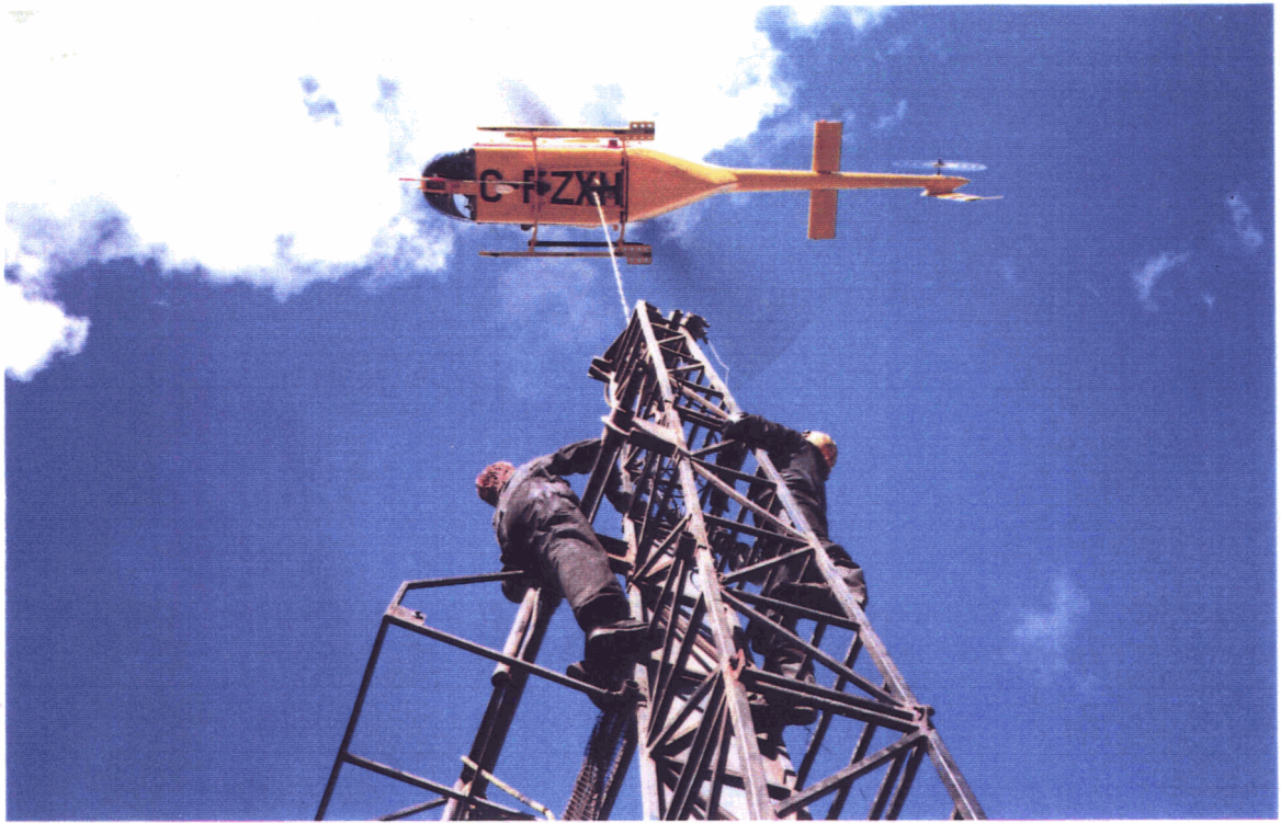
Plate 12: Moving the drill with the helicopter.
