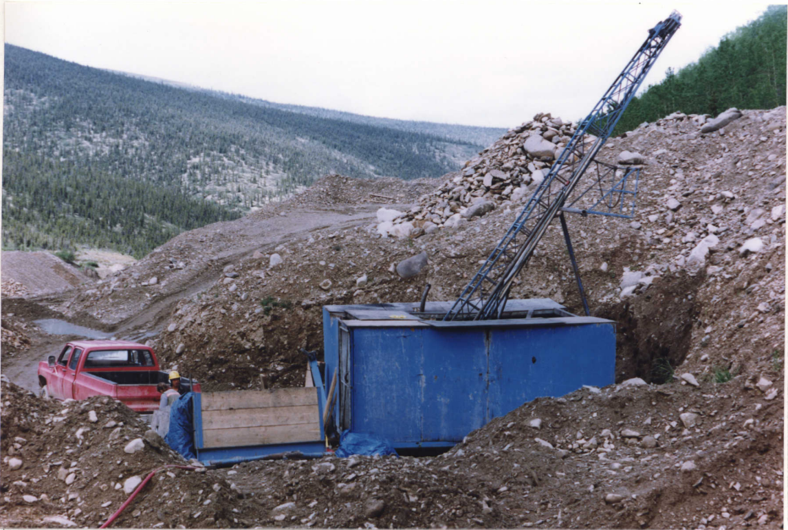
PHOTO 1. DRILL HOLE RWS 89-1 ON SECTION 55+00E SHOWING TYPICAL BOULDER STREWN GRAVEL OVERBURDEN.
