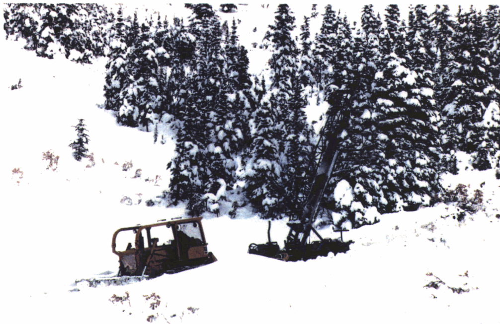
Photograph 8: Moving the drill with the D6 bulldozer, October, 1988
