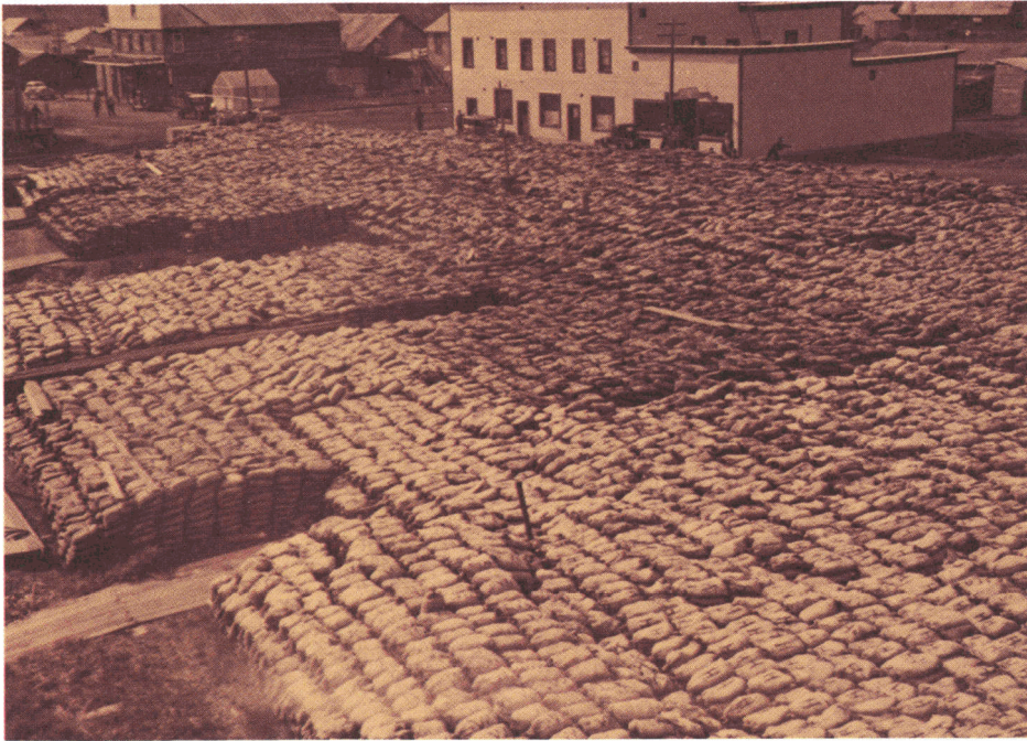
12,000 tons of rich Treadwell Yukon Corporation ore and concentrates stockpiled on river bank at Mayo in 1938 awaiting shipments by stern-wheeler to outside smelters 2,500 miles away.
