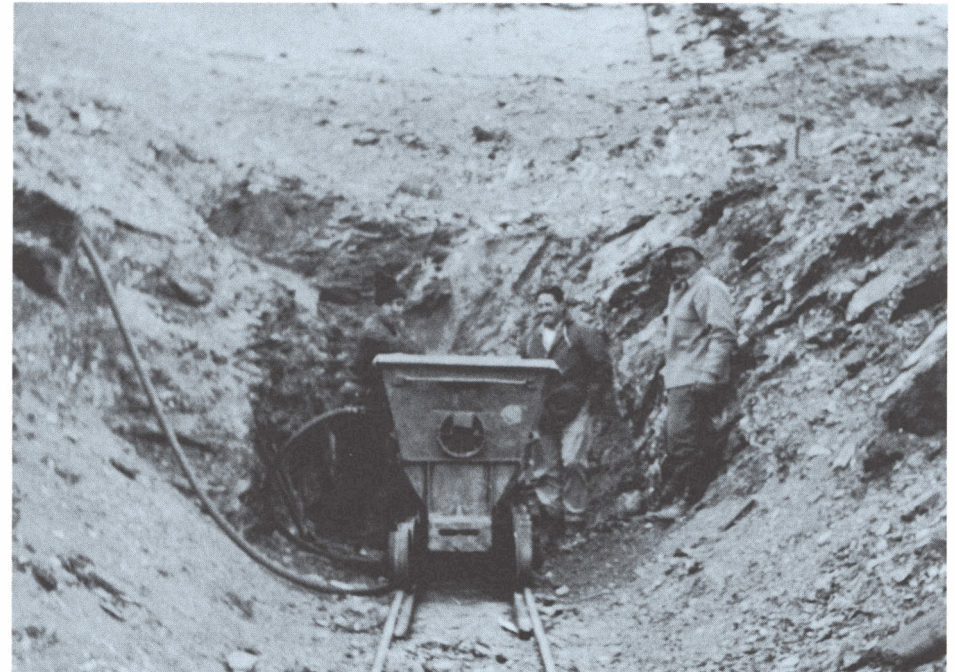
Open cut to adit portal site on Duncan property.
