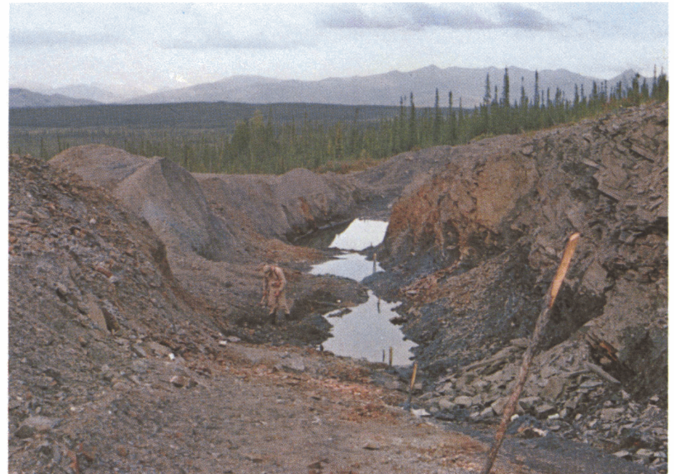
Bulldozer trench on Gerlitzki vein on Galena Hill property.
