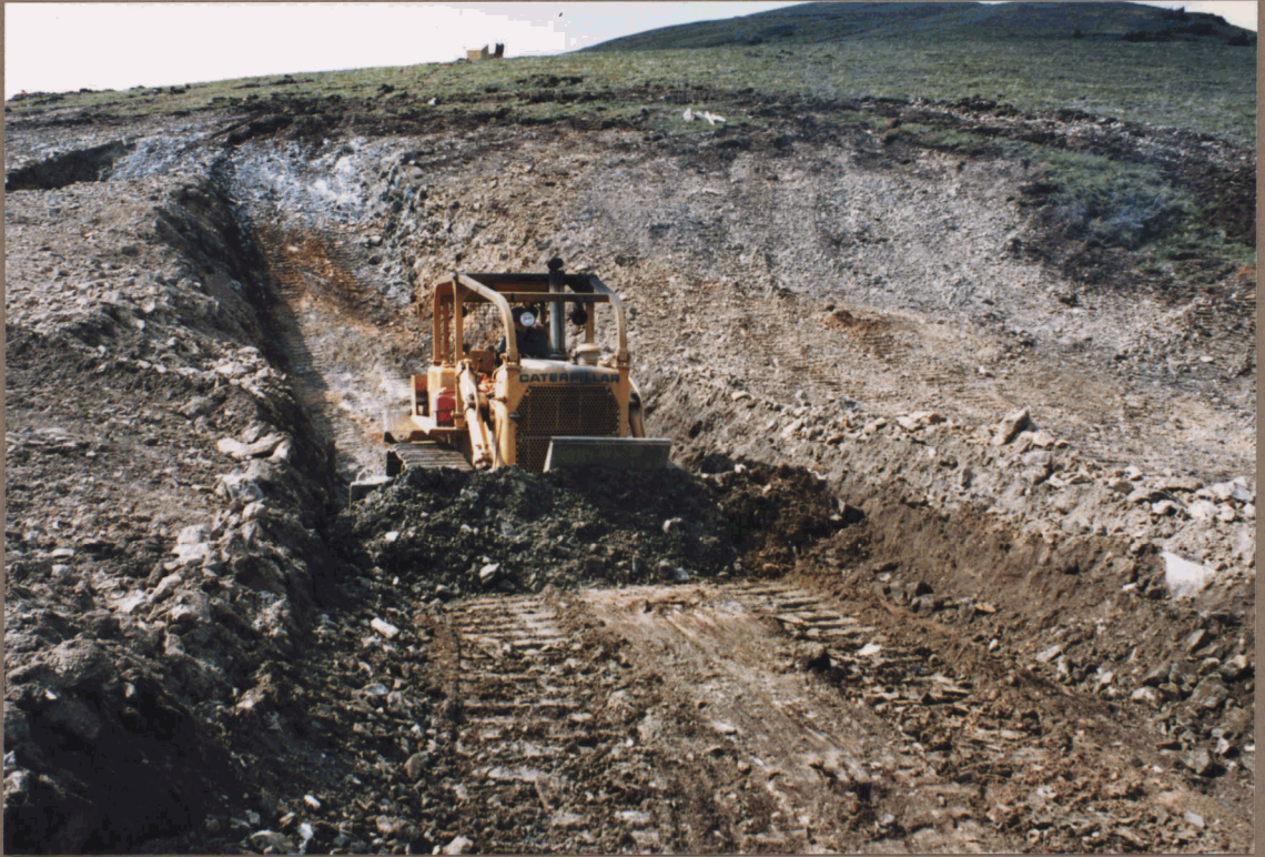
4. Trench number 3, ORO property.
