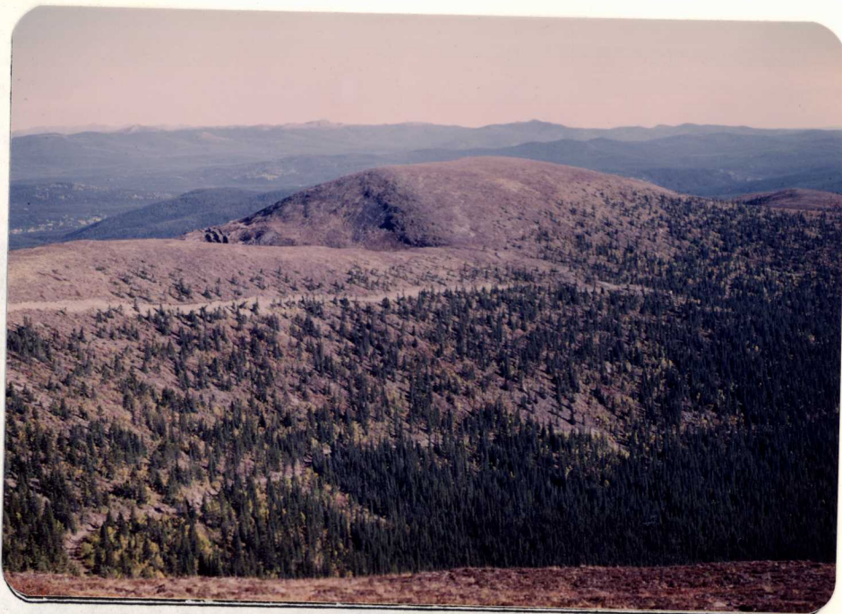
Looking southeast - Access Road - Drill Camp Right Centre at timber line. South Showing stripping 2nd hill.
