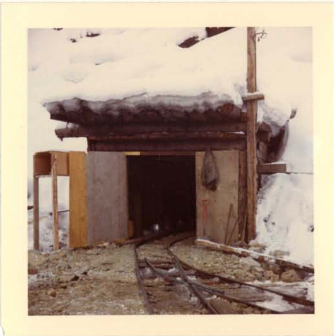
PICTURE #3 - Mine Portal - looking south
