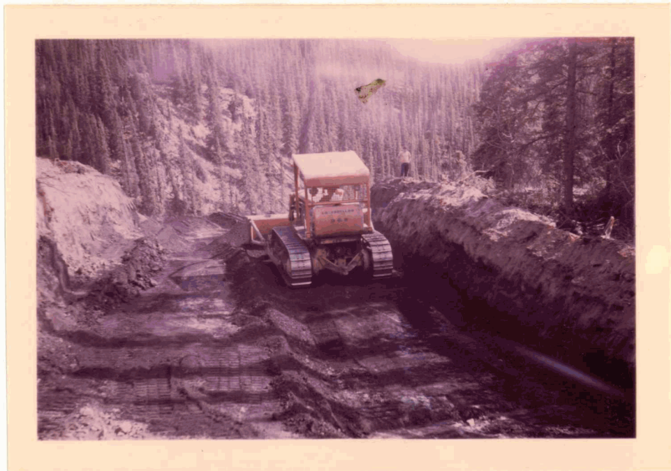
Photo No. 6 - Trenching with D6 Dozer in Pit No. 2.
