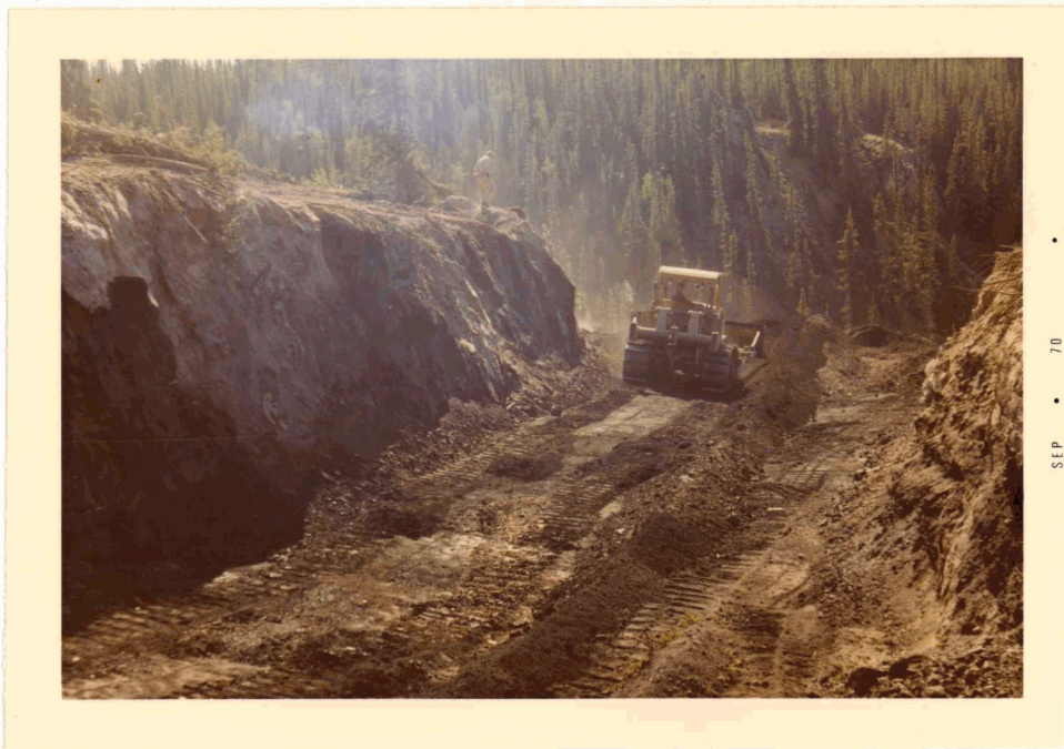
Photo #7. - View of coal outcrop before Pit No. 2 was Trenched. Note excavation centre right believed to be where Cairnes sampled in 1908
