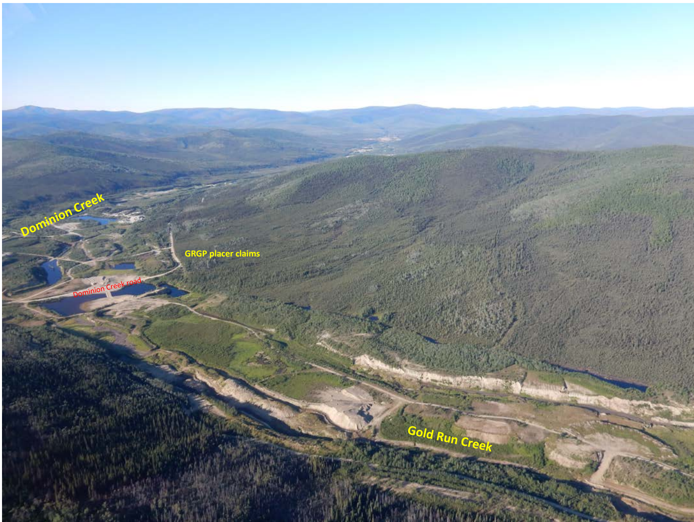
Plate 2 – Aerial view of lower Gold Run Creek at the confluence with Dominion Creek, showing the location of the GRGP claims on the right limit bench. Photo taken July 18, 2018.
