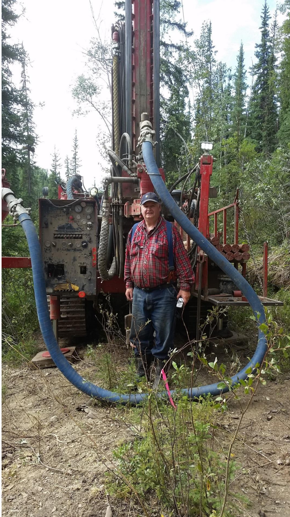
Photo 3 Reverse Circulation Drill Rig on Site
