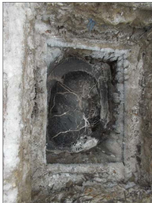
Figure 9. Shaft on opening - February 2013.
