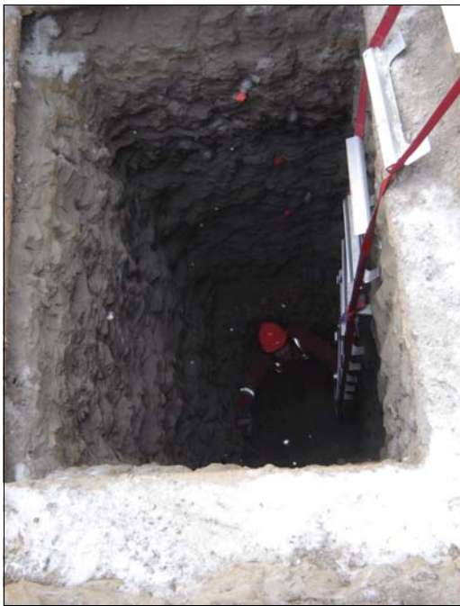
Figure 8. Shaft CC-2 at 19 feet on 17 Mar 12
