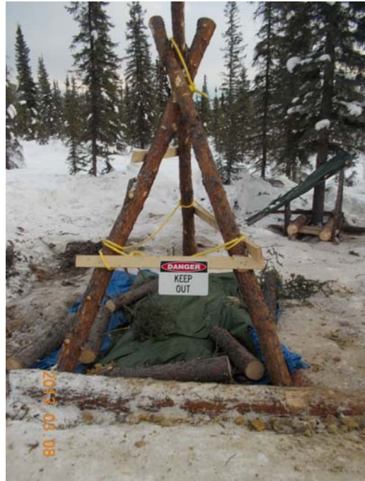
Figure 11. Shaft, covered and ready for final backfill - Mar 2013.
