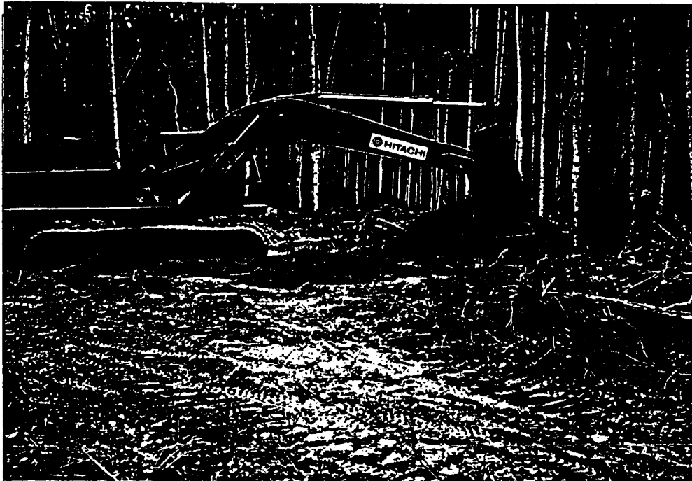
EXCAVATING PITS IN RIVER BANK GROUND
