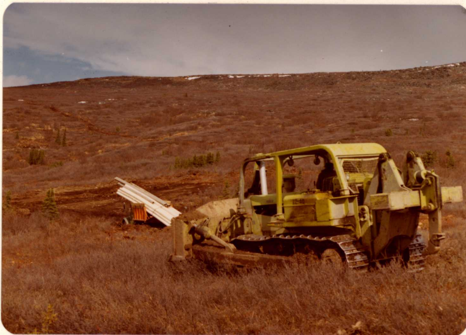
Headwaters of Kenyon Creek as seen from the south. The Terex tractor equipped with ripper was used to dig test pits. May 1976.
