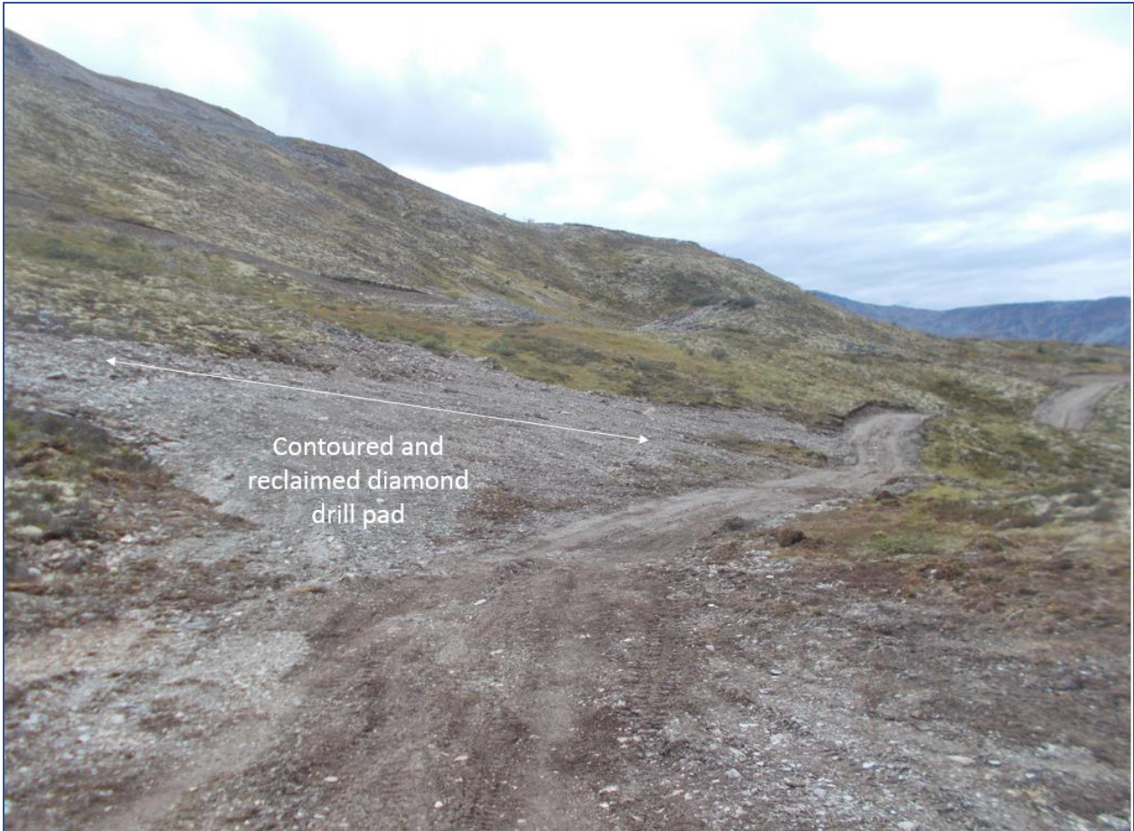
Figure 22: View to west on reclaimed GC1802 drill pad.
