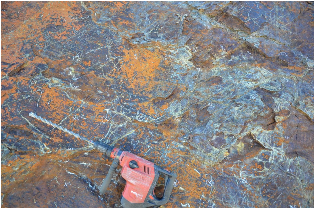
Illustration 10: Drilling grid marked in white China marker
