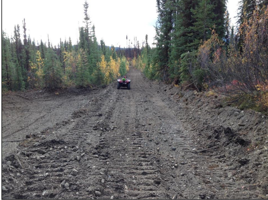
Photo 2 – Road construction on the Plata property
