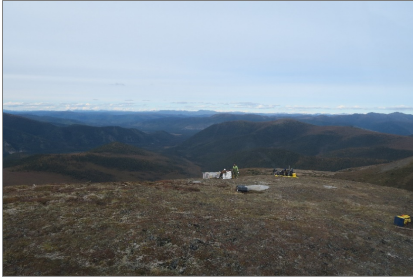
Figure 11: RAB drill mobilizing at the Charon North target at the Pluto Property. Photo taken on August 28 th , 2017.
