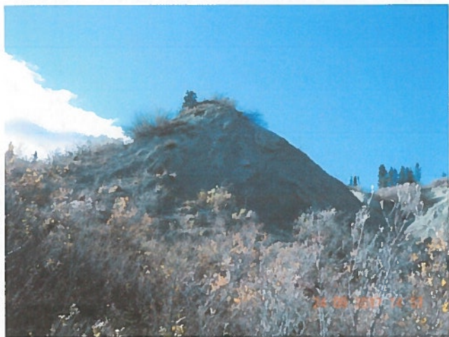
Picture 6 - Visible ground fractures
