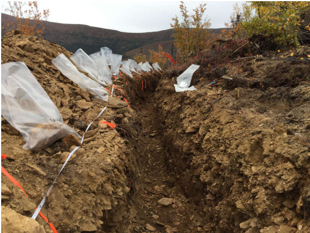
Photo 2: Trench 3 looking north.
