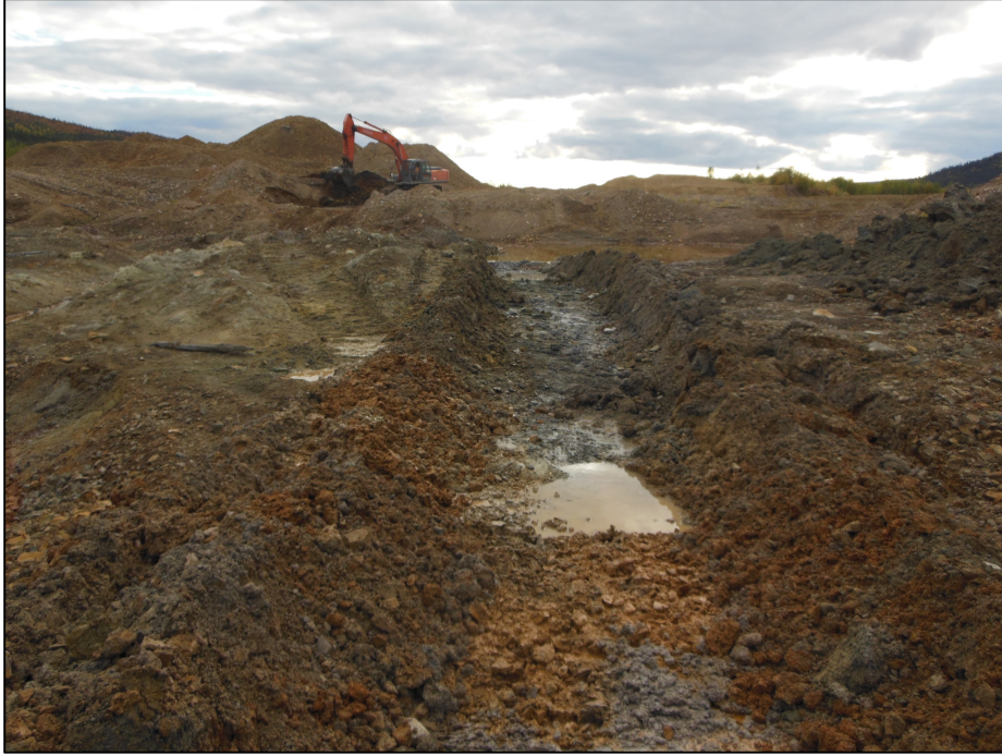
Figure 9. Shallow trench in altered andesite bedrock at station RH17SM022.
