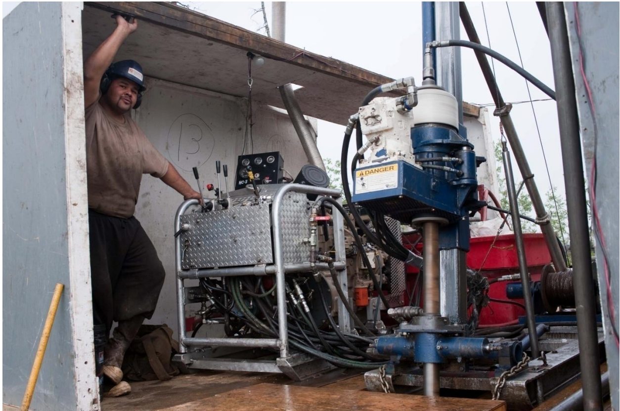
Figure 45 Peak Drilling Hydracore 2000 diamond drill rig.
