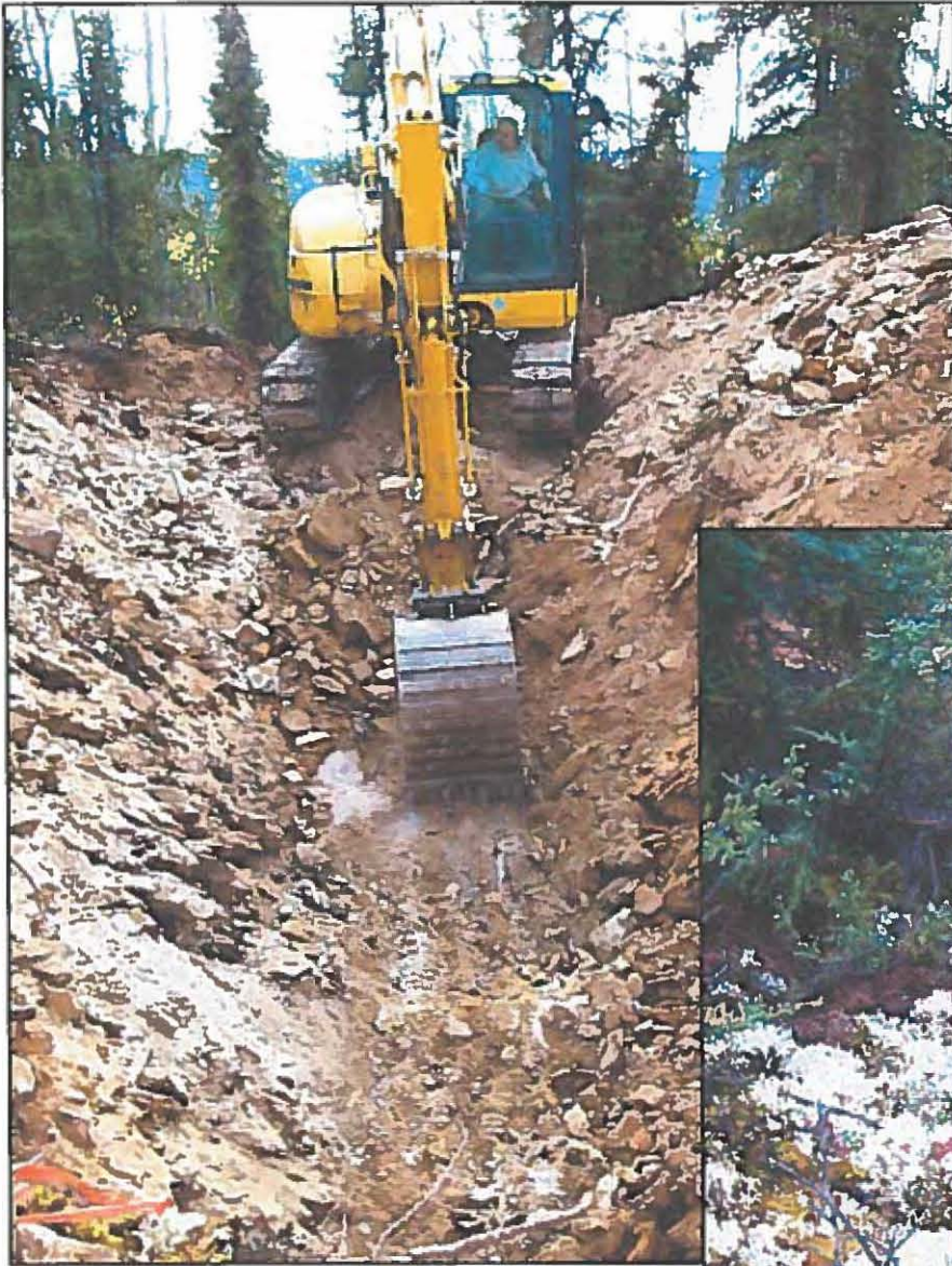
Left: Trenching above Coarse Gold Creek with Komatsu hoe
