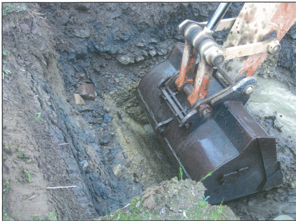
Figure 7. Above. Trench 09-01 at 0+01m showing placer gravels overlying altered (yellow –tan collar) altered andesite. Bucket just under 1m wide.
