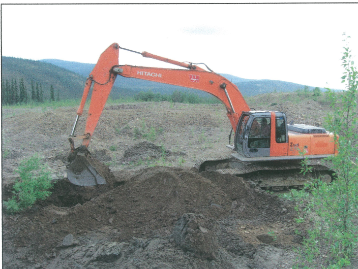
Figure 6. Mike McDougall excavating Trench 09-01.
