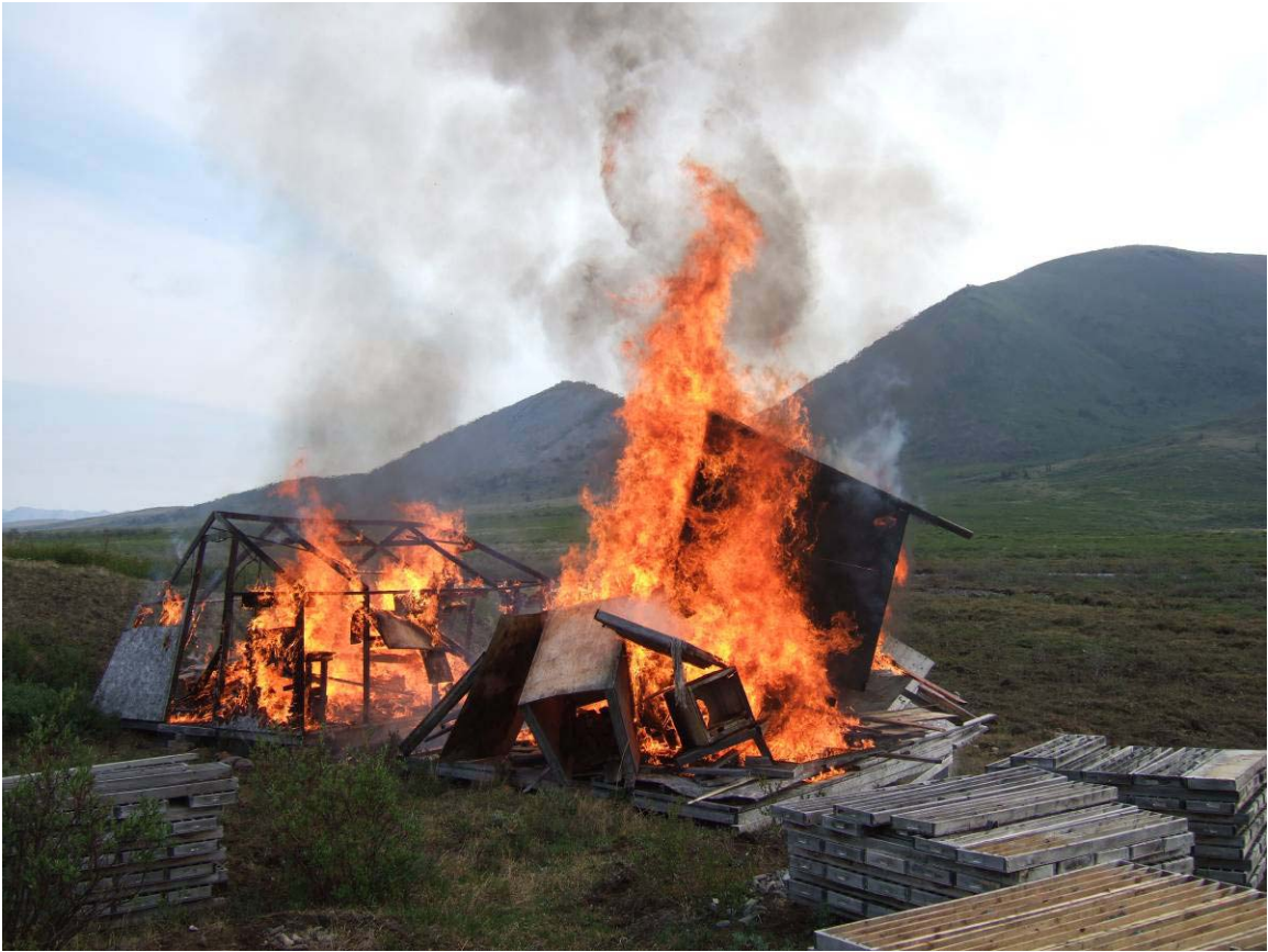
Burning of former Pyramid Valley drill camp structures
