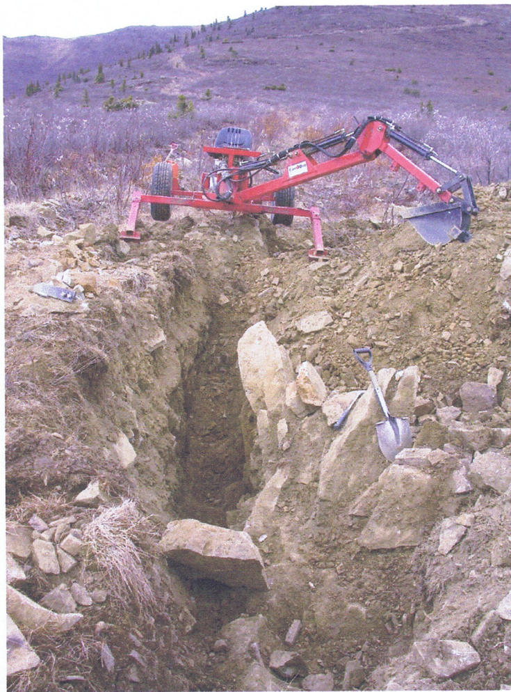
Can Dig Excavator Digging Black Fox Trench
